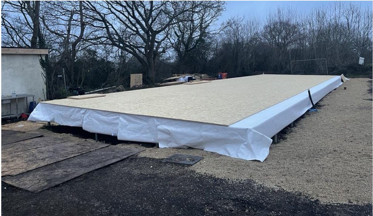
Completed works on the foundation with 150mm Celotex insulation under floor, with Tyvek firecurb membrane installed (White sheet below OSB floor).
